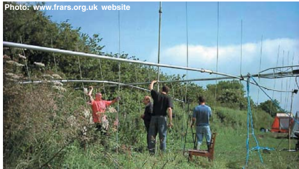
Members of the Flight Refuelling ARS putting together their monster 6m and 4m antennas.
